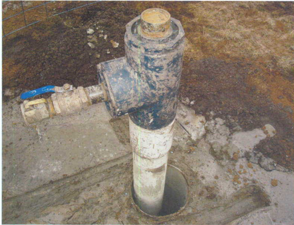
Photo #6: Completed hole, west site
